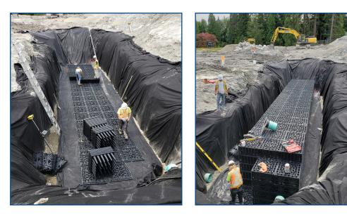
The project began with EcoBloc Maxx base plates laid at the base of the site bed and secured with connector pieces. Blocks were then stacked and connected up to five layers and finished further endplates and pipe connections. Pipe adapters were used to secure the pipe connections in place. The structure was then wrapped with 8 oz. geotextile and an inspection port was secured. Finally, the site was backfilled evenly with gravel.
